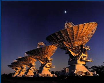
ATCA : 6 antennas each 22 m in diameter
