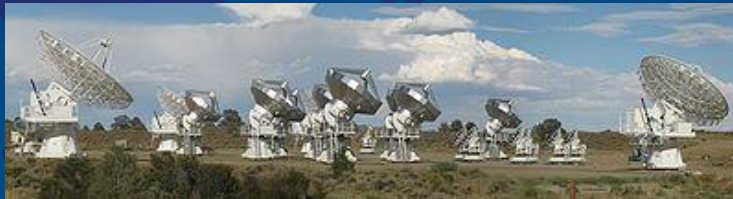
CARMA • 6 Antennas each 10.4 m. in diameter. (OVRO) • 9 Antennas each 6.1 m. (Hat Creek) • 8 Antennas each 3.5 m. in diameter. (SZA)
