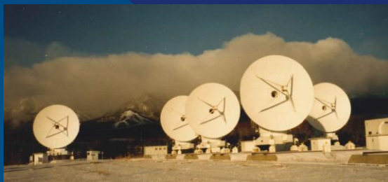
NRO: 6 antennas each 10 metres in diameter
